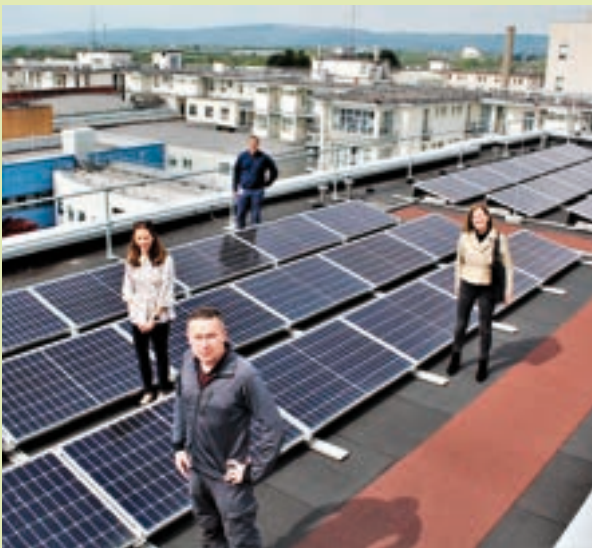
Pictured at the bank of solar PV cells on the roof of the 60-bed block at UHL; Kevin Mahoney, Rachel Keating, Clodagh Hanratty and Niall Joyce
